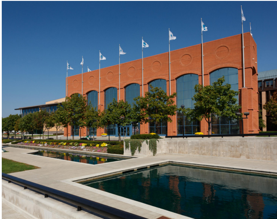
NCAA Hall Of Champions; Indianapolis, IN; UltraPly™ TPO and Metal Wall Panel Systems
