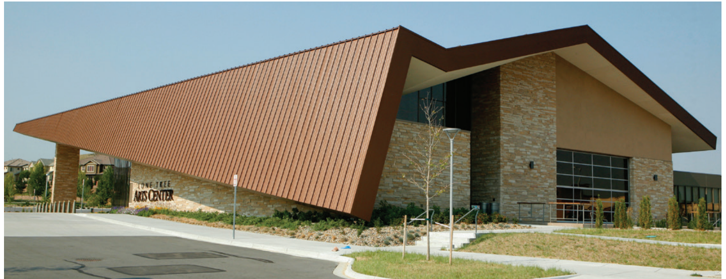
Lone Tree Cultural Arts Center; Lone Tree, Colorado; RubberGard™ EPDM and Metal Roof System
